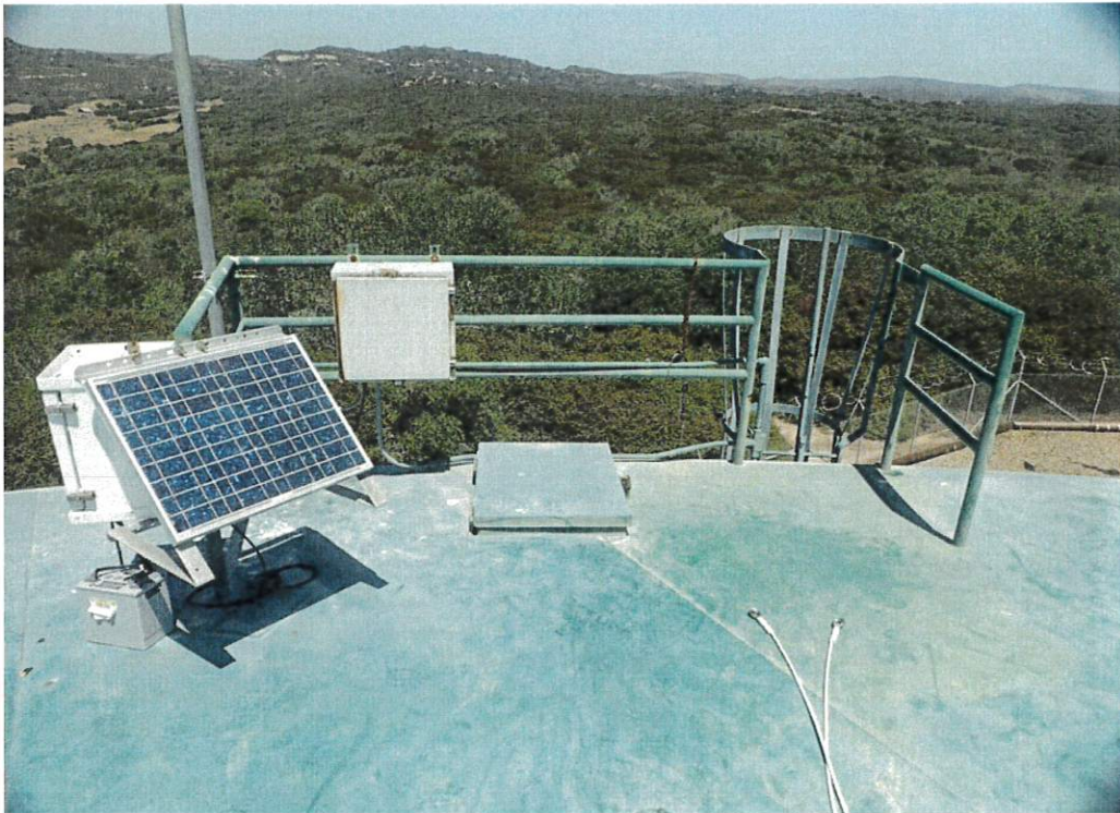
The photo above shows the roof hatch area with limited guardrail. Tie off cables are present (Installed by ATS personnel) but no self closing safety gate has been installed so full time tie off for personnel is required.
