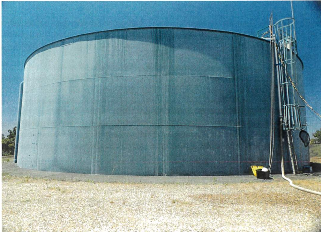
Overall view of the tank.
