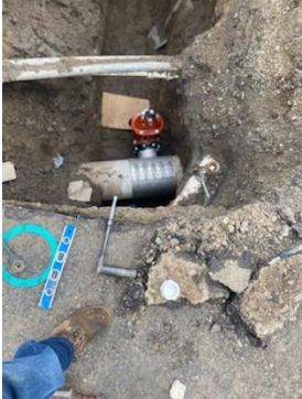
Site prepped/ready for Surge Tank Installation:
