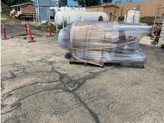
Concrete slab to be poured between orange cones / surge tank wrapped for protection:
